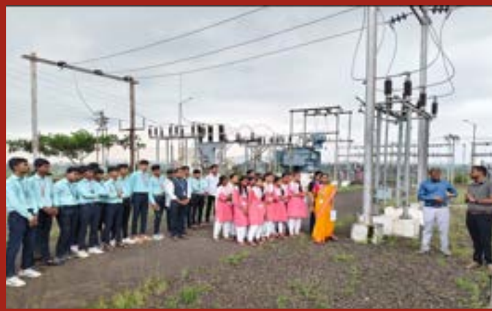
Discussion between students & assistant engineer on working of substation
