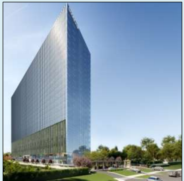
The BIM model of a building in India GFM Godrej Projects KP and Bangalore
