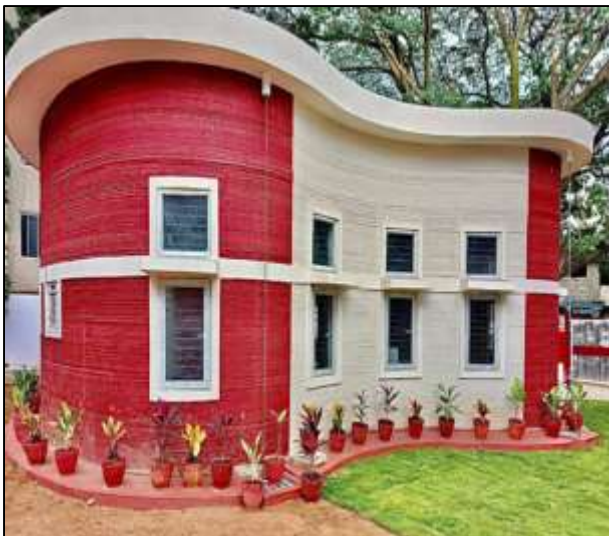
The first 3D printed building in India Cambridge Layout Post Office , Bangalore
